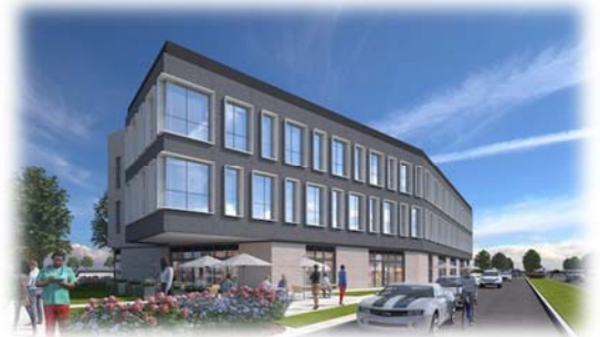
One Lawndale Community Care & Surgery Center at Ogden Commons
